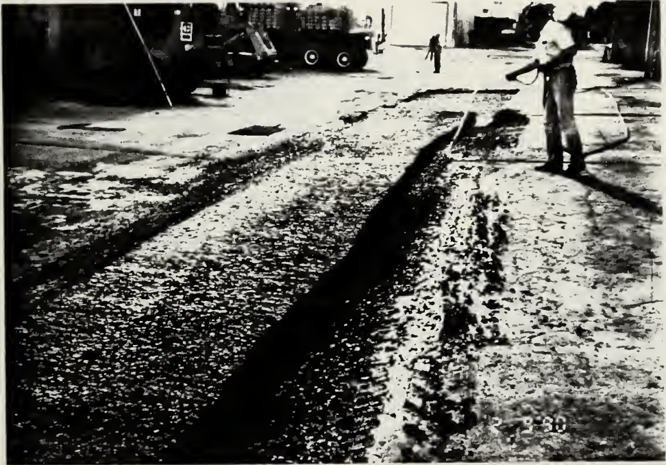
Figure 2.21 Additional Water Placement
